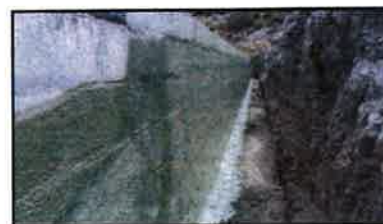
READY FOR BACKFILL
